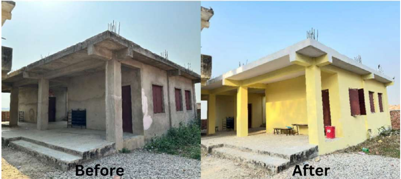
Before and after the colouring school building wall
